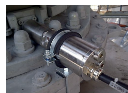
Coupling unit with bushing tap adapter
